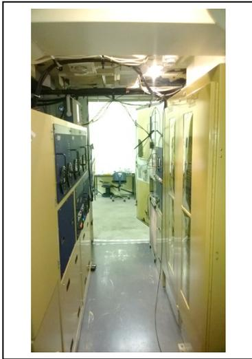
Fig. 6. Solid-state modulator installed in a shelter
